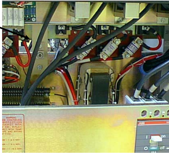
FIGURE 3.7.1 OUTPUT CONTACTOR (CUSTOMER LOAD WIRING DETAIL)
